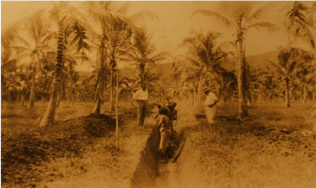
Figure 1: 'Showing the completion of a conserver drain', Solomon Islands, 9th December 1924. UARM, SDC/3/2/11
